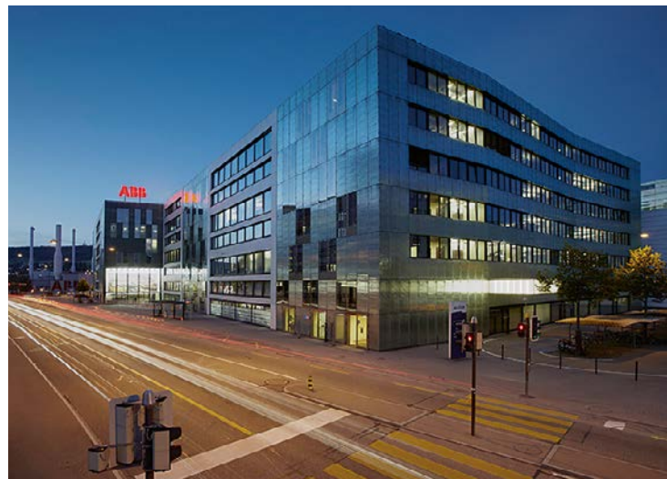
ABB Power Tower, Baden
